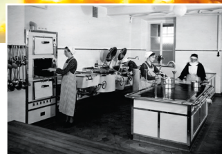
Cooking installation in Kloster 1960
